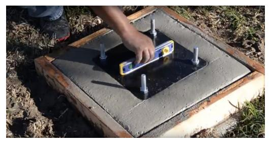
Once completely smooth let the concrete cure. This can take up to a week. Consult the instructions on the concrete bag for curing times and directions.
